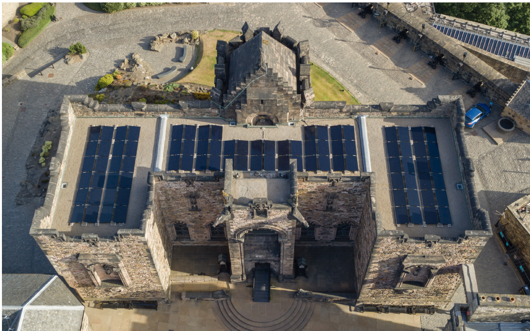
Figura 1. Paneles fotovoltaicos en el castillo de Edimburgo, Patrimonio Mundial. Fuente: Historic Environment Scotland (HES). National Collection of Aerial Photography (NCAP)
